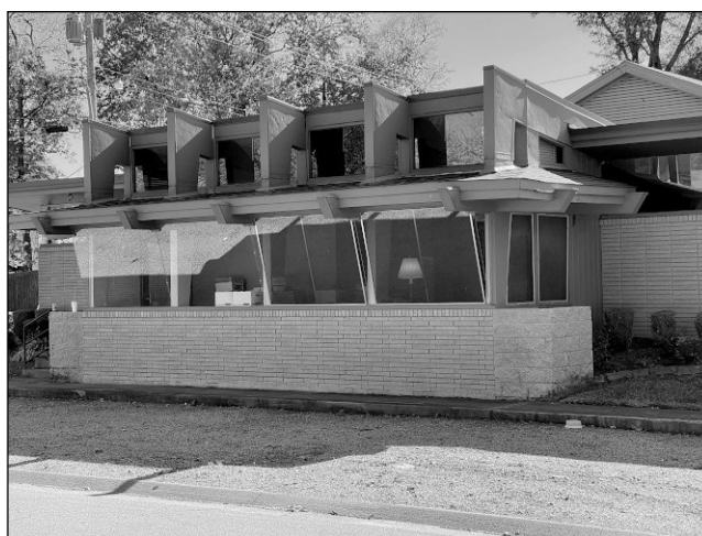
DR. BOST BUILT THIS CLINIC BUILDING in Fort Smith and moved in in 1958.
