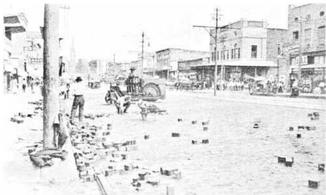
Replacing wooden blocks on Garrison Avenue after a rain. Courtesy Bernice Cole.
