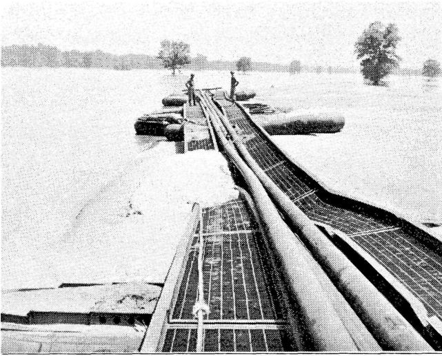
Restoration of water service to Fort Smith across flooded Arkansas River, May 1943. Courtesy Fort Smith Chamber of Commerce.
