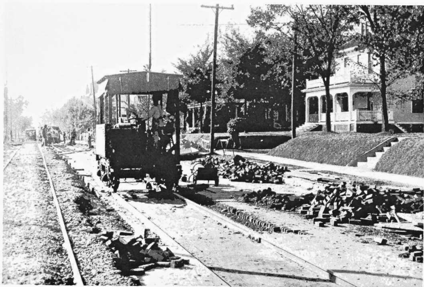
BONDING and CONCRETING SOUTH 21st and E STREETS
