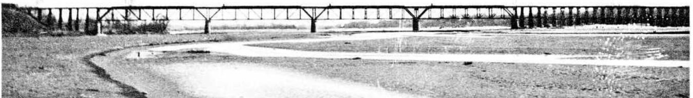
The troublesome South Canadian River is only a trickle in this view of the bridge. The trestle that replaced a washout of the high curved embankment is visible on the right. J.B. Fink Collection.
