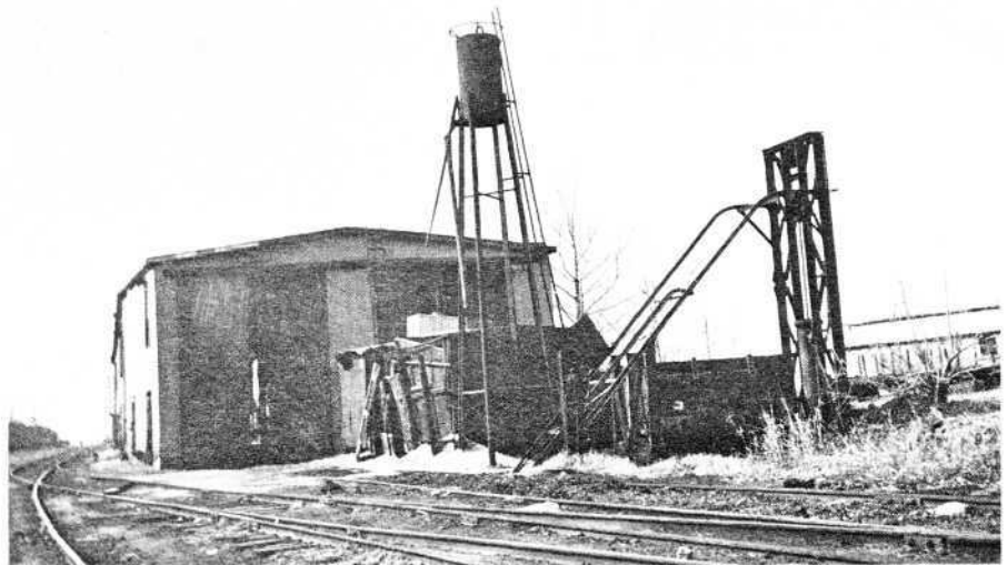
Frame and stucco boiler shop erected about 1916, one block south of "D" Street, with tools and equipment to permit boiler repairs, fabrication and installation of new fireboxes to F.S. & W. locomotives. The tall object in the center was the sand tower and the steel tower to the right was a hoist to draw cinders out of a pit up the inclined rail to dump them into a gondola car. J.B. Fink Collection, University of Oklahoma.
